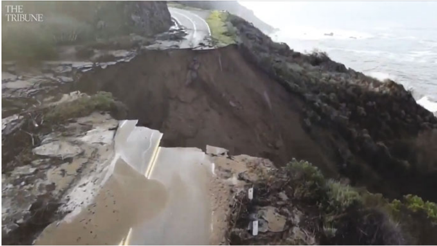
Fig. 7.30 Landslide along California's Highway 1. (Photo credit San Luis Obispo Tribune)
